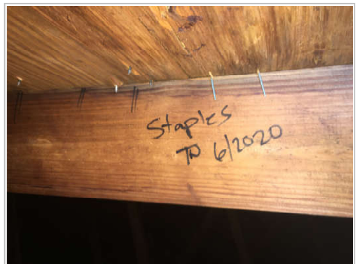
Stapled Roof Deck
